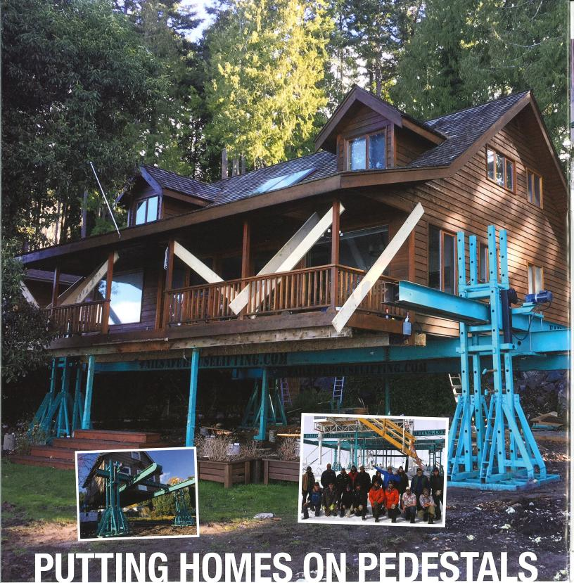
FailSafe adds security during foundation repairs/replacements
